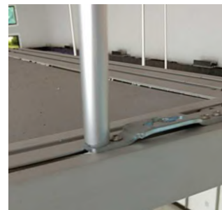
Suspended CLOUD MEDIA FRAME by rigid poles
